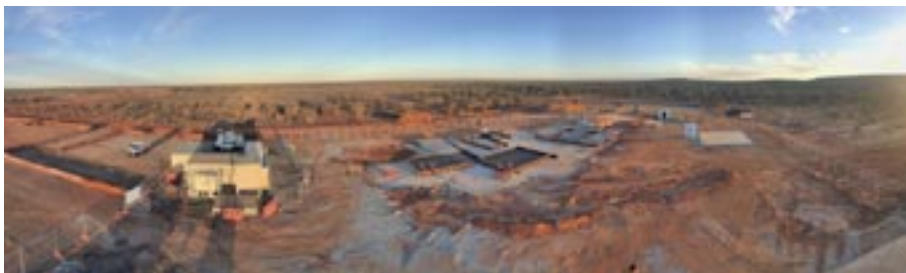
The foundations for the fans to be installed at St Barbara's Gwalia underground gold mine will consist of over 1,500 t of concrete and 300 t of steel
