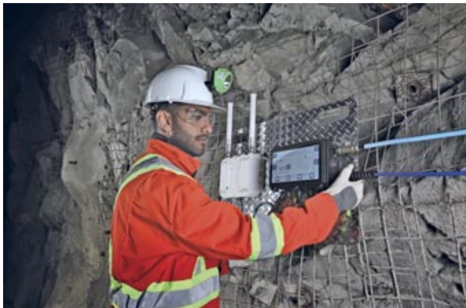
Maestro Digital Mine Plexus PowerNet with Cisco WAP at Borden gold mine
