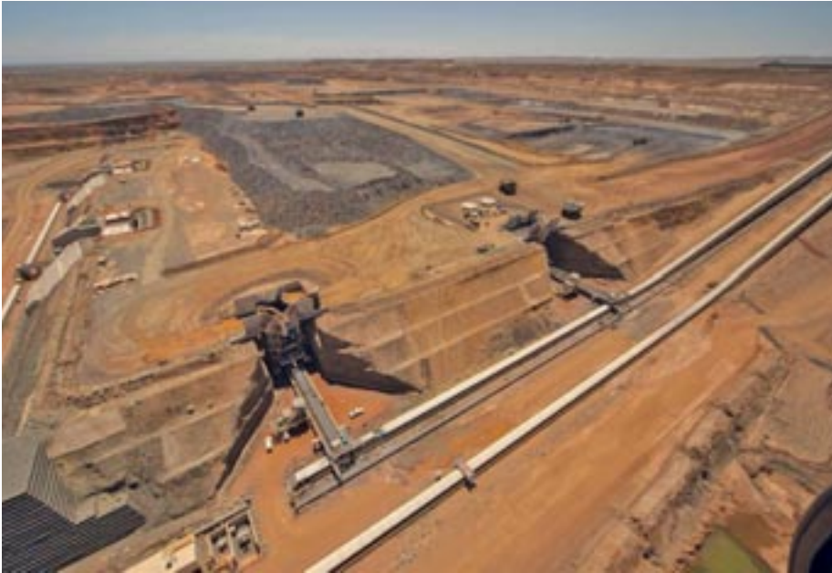
At Citic Pacific Mining, Huawei's eLTE solution implements seamless Wide Area Network (WAN) coverage for truck dispatching, and eliminates the need to routinely relocate base-stations
